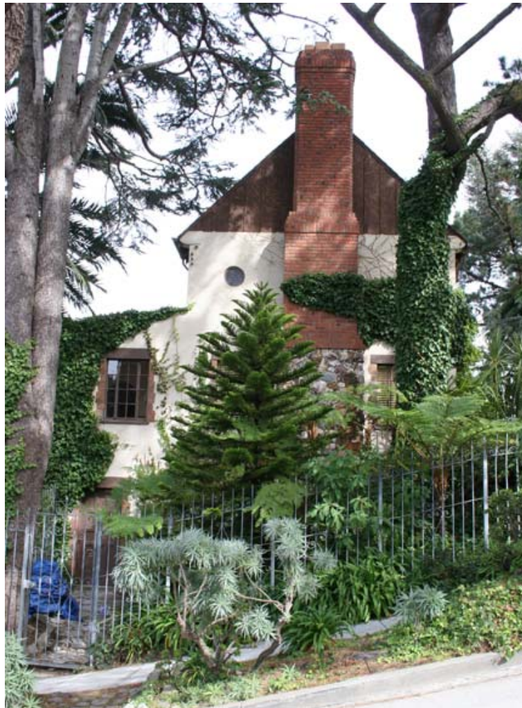
Figure 5. West façade, looking east. (Source: Bruce Tomb)
