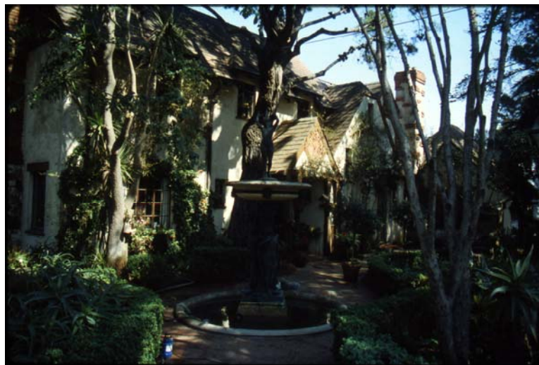
Figure 19. 3690 21 st Street, entry courtyard and front façade, looking northeast. (Source: San Francisco Public Library)
