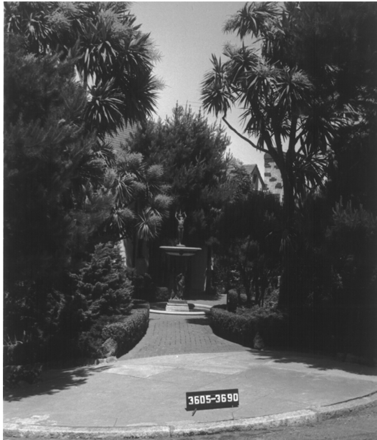
Figure 20. 3690 21 st Street, entry courtyard from the southwest, date unknown. (Source: San Francisco Assessor)
