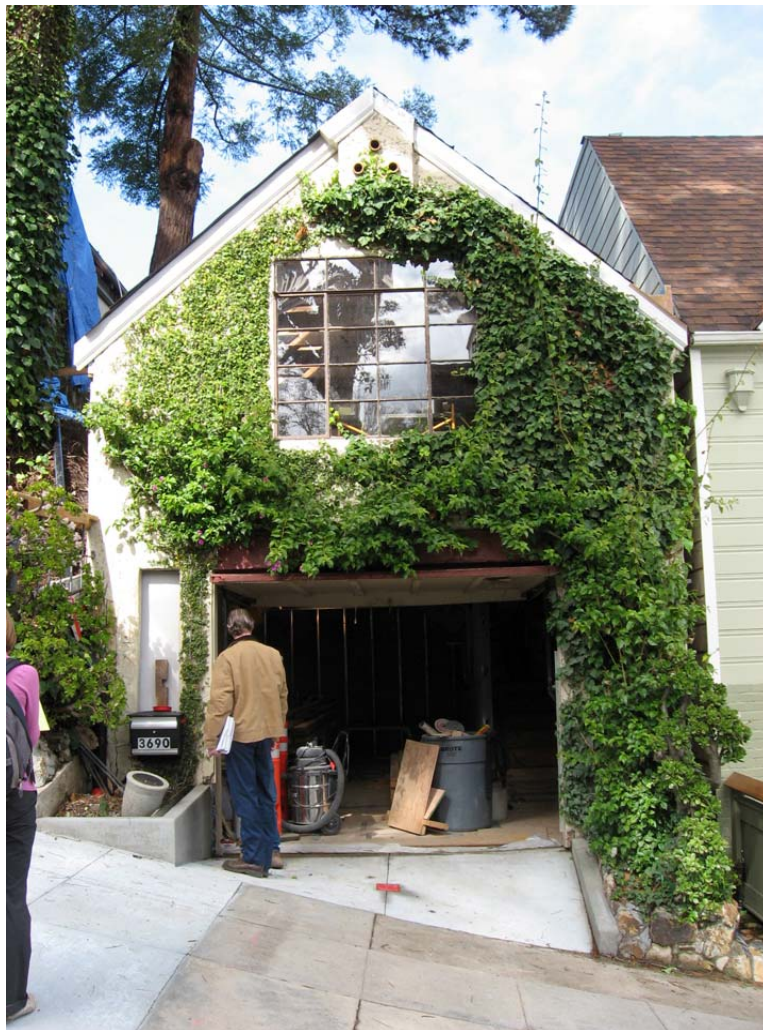
Figure 10. (left) Primary façade of garage from 21 st Street. (Source: Page & Turnbull)
