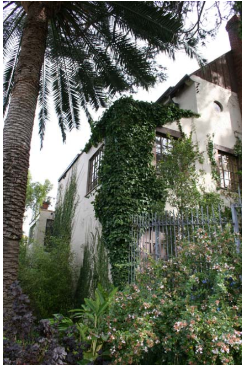
Figure 8. Northwest corner of house, showing north façade at left. (Source: Bruce Tomb)
