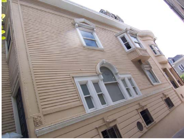
Figure 4. West elevation, from north
