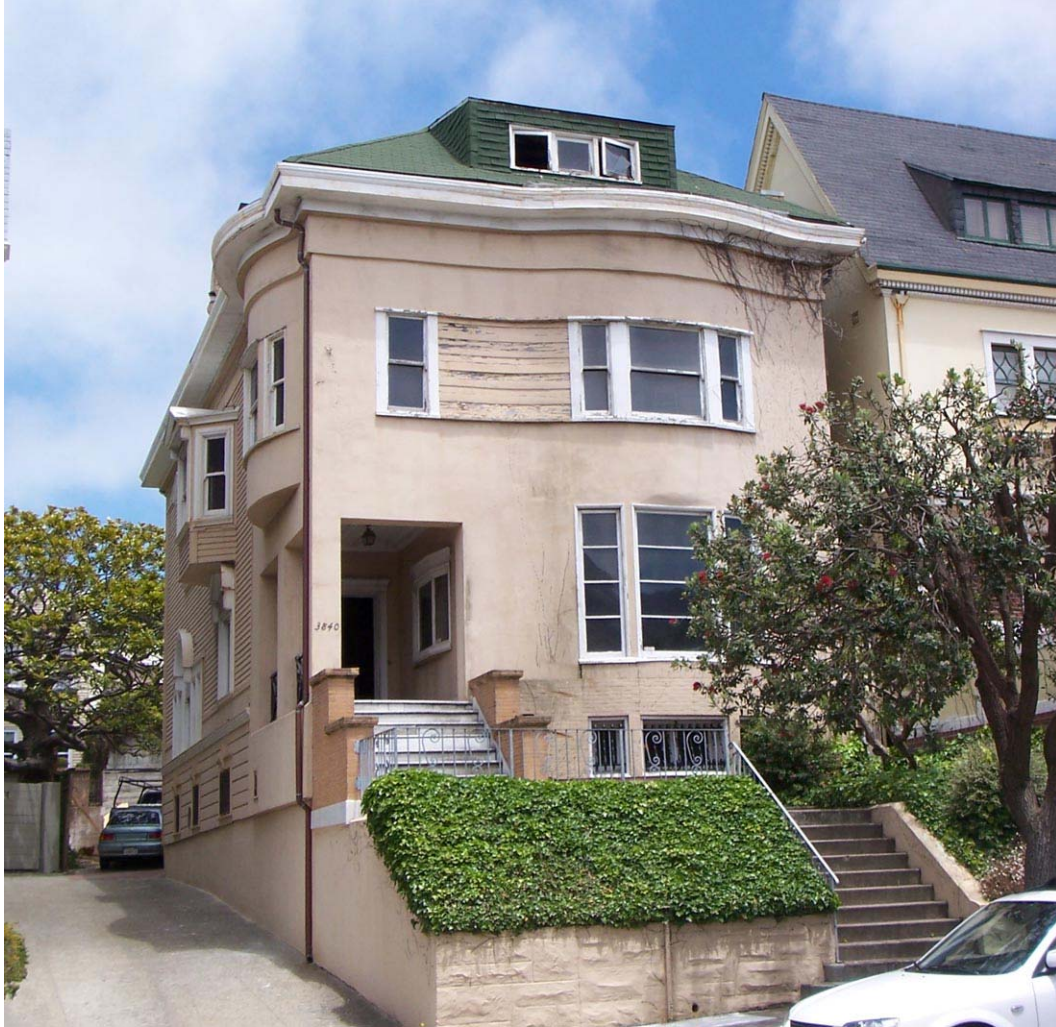
Figure 2. 3840 Clay Street, from south
